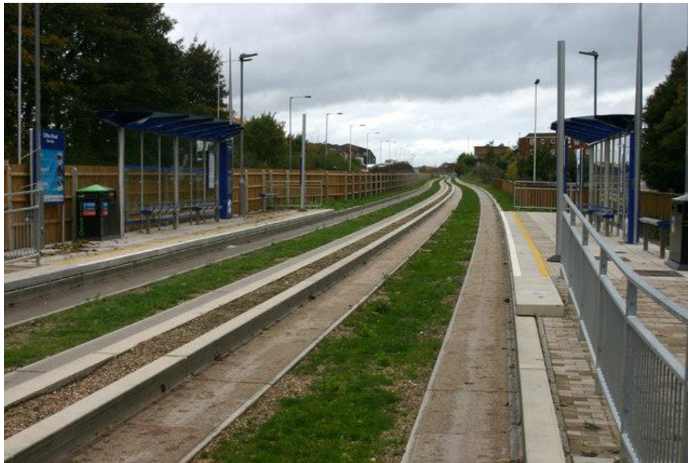
Luton Dunstable Busway has a concrete track to guide conventional buses which are fitted with special guide-wheels
